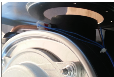
Figure 14. Flue fuse
