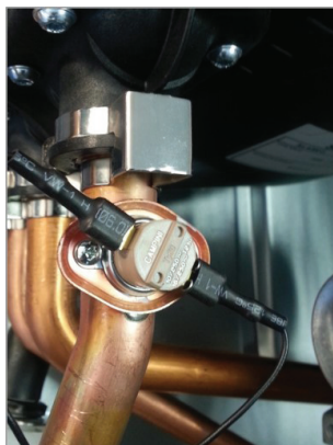
Figure 16. Limit thermostat
