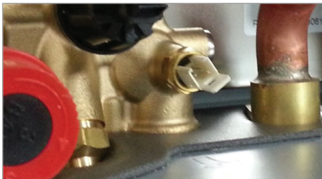
Figure 21. DHW temperature sensor
